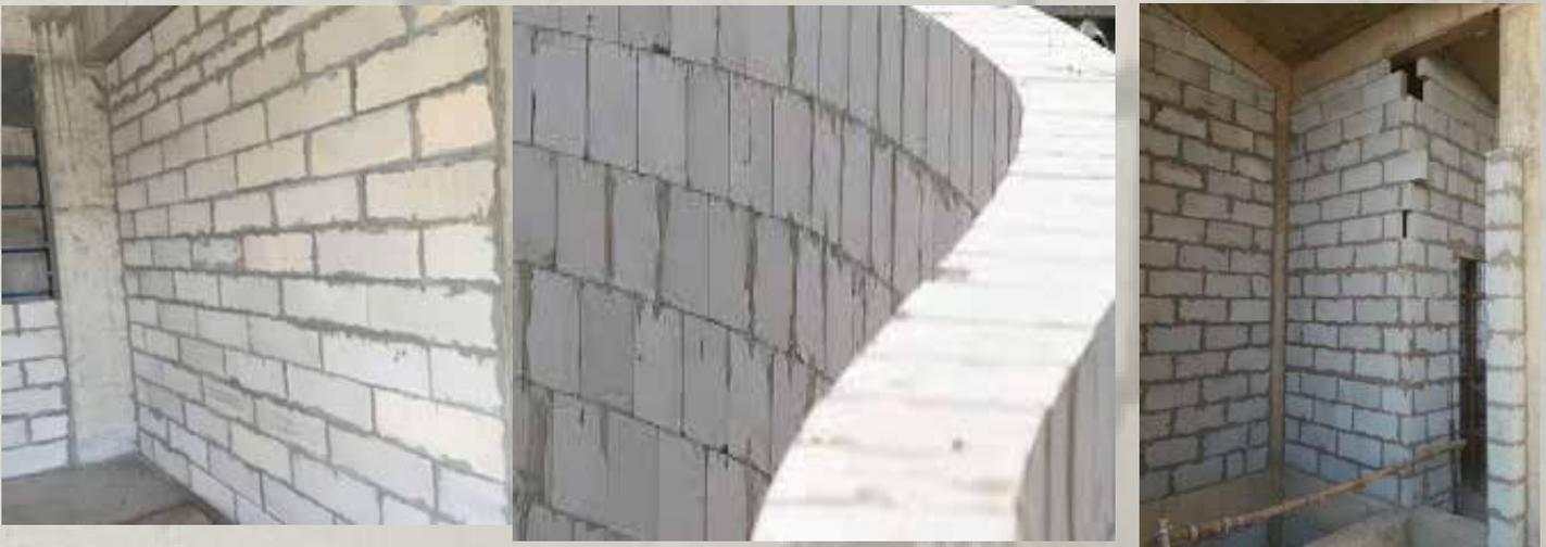
**ECOCON Superlightweight Blocks (less than 275 kg/m<sup>3</sup>)** can be perfectly applied as filler (hoardy) blocks for pre-cast panels production. The perfect thermal insulation of superlight blocks allow to avoid usage of expensive and fire dangerous polysterene.
