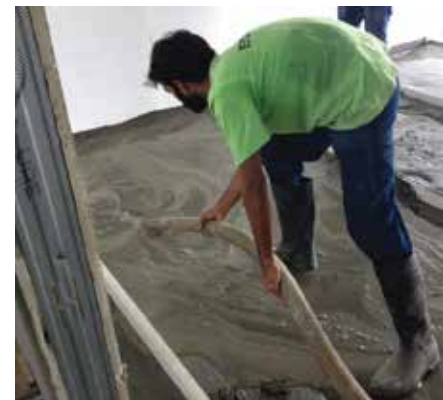
Pos. 10 Filling of ECOCON screed
