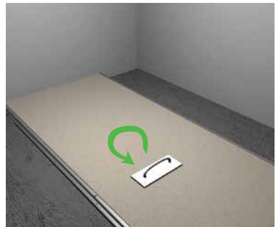
Pos. 14 Finishing of ECOCON screed with darby
