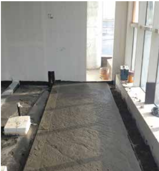
Pos. 13 ECOCON screed after second levelling
